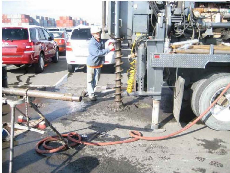
Photo 1. Drilling boring SC-1.
